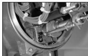
Fig. 10.1 Limit Switch Shaft in Switch Mech
